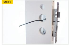
Fit the morice lock to the door. Take care not to trap the cable between the mortice lock and door.
