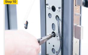
Check correct operation of the throw bolt with pliers.
