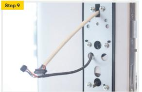
Fit the mounting plate onto the inside of the door to hold the back body in place. Fit the cables through the mounting plate slots. Screw the plate to the door.
